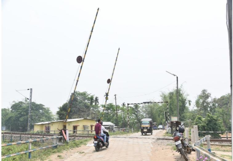
boom arrangements have been provided at 10 LC gates across Kathiawar, Rangia and Tinsukia Divisions of the zone. Sliding booms enhance visibility and physical obstruction at LC gates, significantly improving safety for road users during train movements. A total of 582 nos. of sliding
