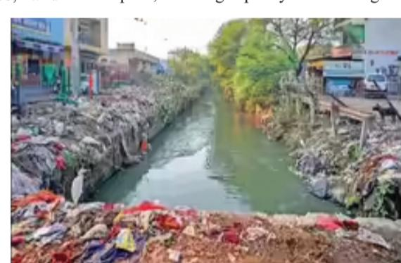
While most of leg-II is covered, the stretch in Ashok Vihar remains an open brick-lined drain. Several portions have partly collapsed, reducing capacity and slowing
