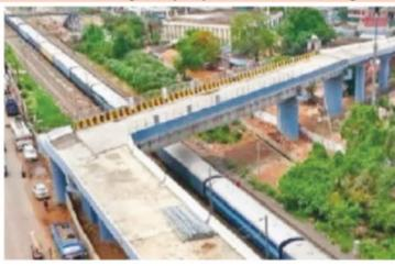
almost 90 degree turn. If the vehicles turn at this angle, they may hit the wall of the bridge or may hit vehicles coming from the front. The Railway overbridge has been built at a cost of Rs 18 crore bridge was under construction, the Railways had objected to this 90 degrees turn.
