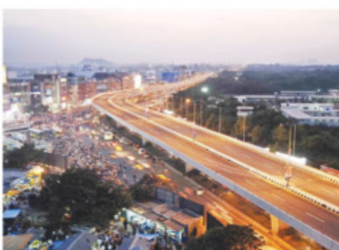
Traffic going clockwise will travel in a series of underpasses while traffic going counterclockwise will use a series of flyovers.
