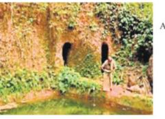
water source, and reviving them will help increase the groundwater level."Surangas were traditionally used by farmers, as many of the tunnels provided water during the summer. A Suranga is essentially a tunnel carved into a laterite hill that allows water to seep through and collect at the other end. Kasaragod is one of the districts in the state that faces acute water shortage in the summer.
