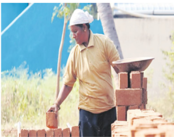
illegal brick kilns in Thadagam valley, which were operating without any statutory approvals, applied for consent to operate
