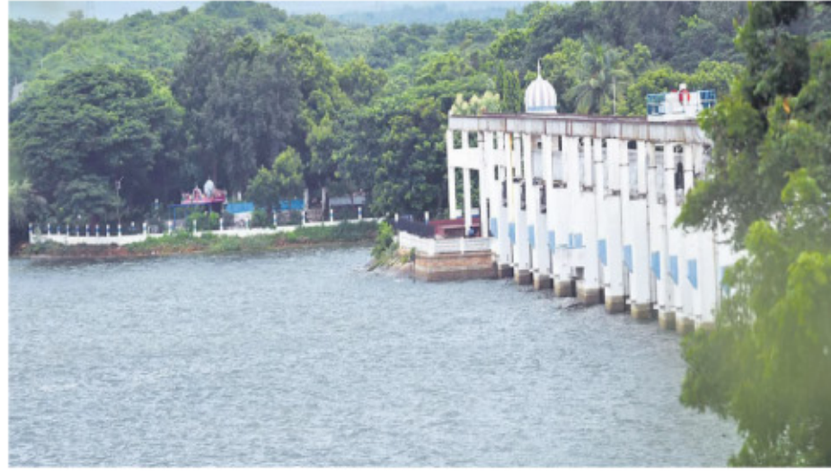
detailed design and drawing. We are yet to finalise the project cost, but it is estimated to be around Rs 100 crore. WRD plans to complete the project in four to five years,” a
