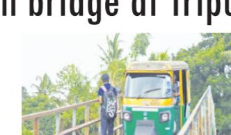
constructed by the irrigation department in 1999. It's in a dilapidated condition now, with gaps appearing at one end. The hand railings have corroded. It's slippery during the rainy season, and a small mistake can land a vehicle in
