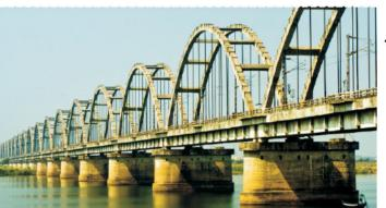
Godavari River. Standing tall on 28 piers, the 2.7-km-long stretch is shadowed by stunning parabolic arches,
